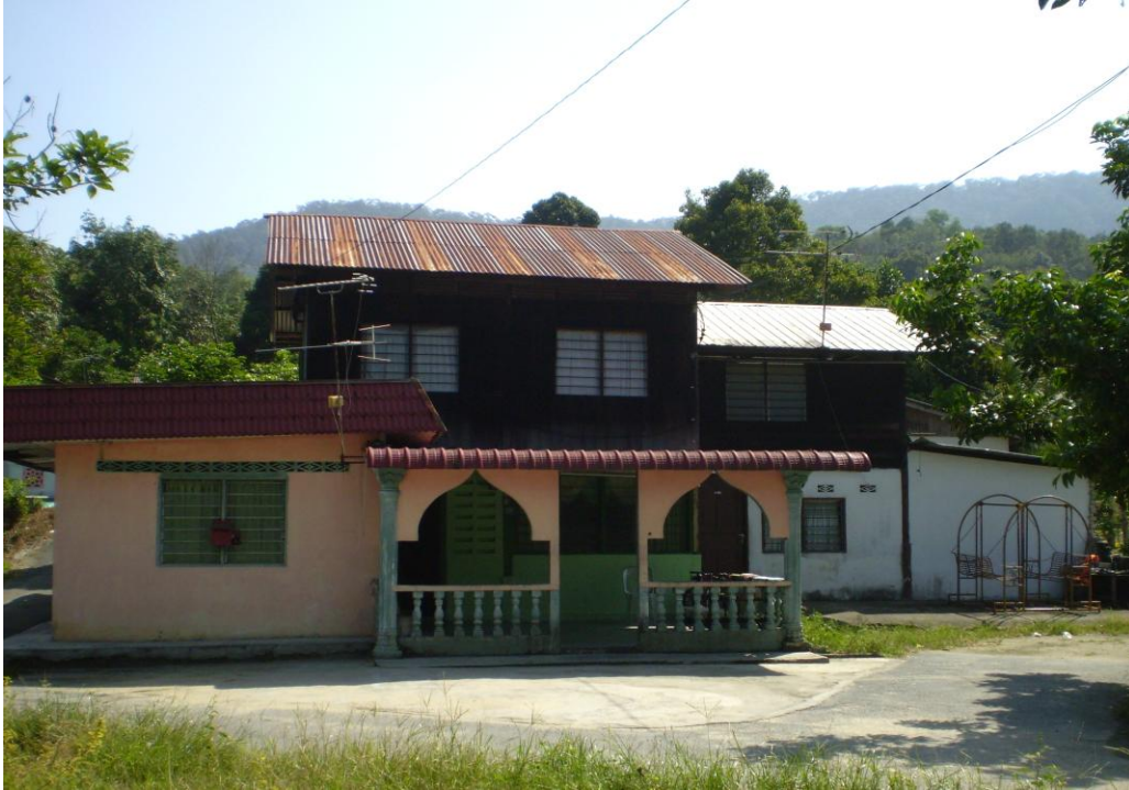
A house in Penang, Malaysia.
