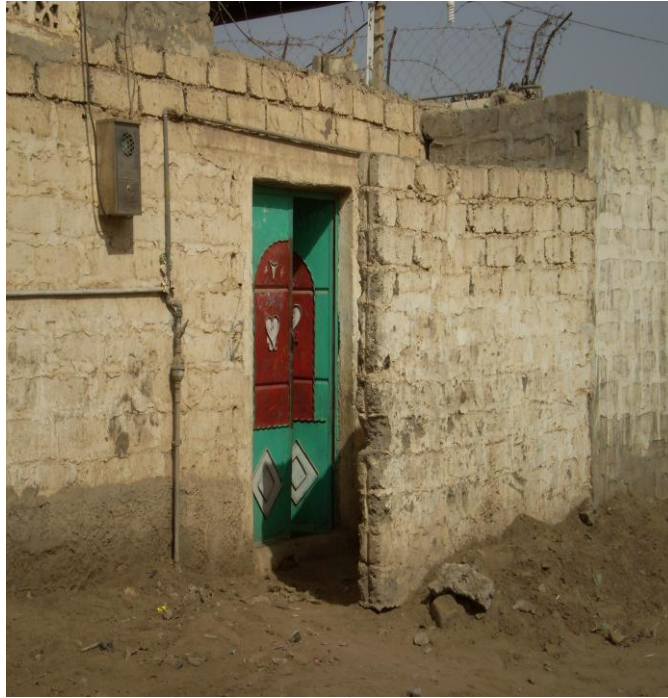
A wall placed just outside a front entrance for privacy protection in a house in Zabid, Yemen.
