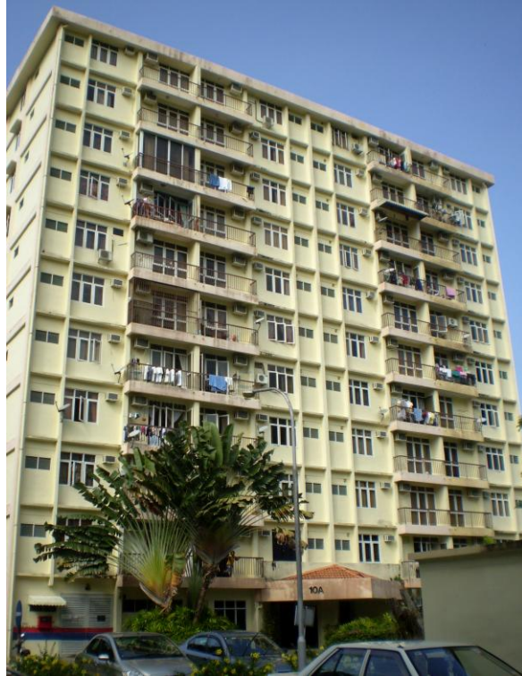
An apartment building in Penang, Malaysia.
