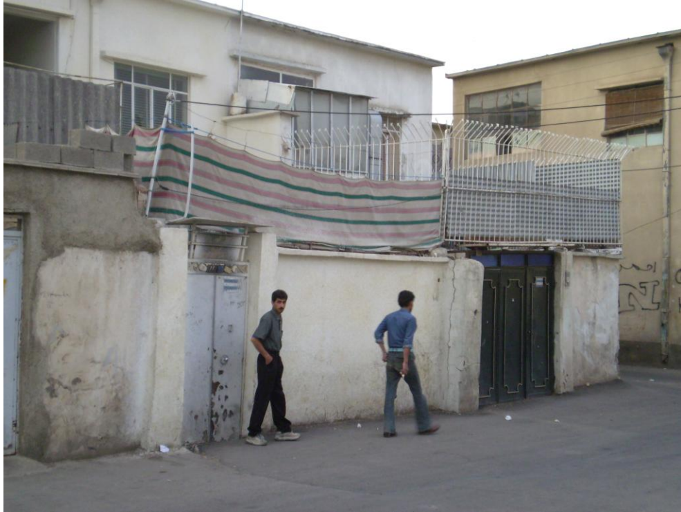
Crudely screened courtyards in these two houses in Shiraz, Iran.
