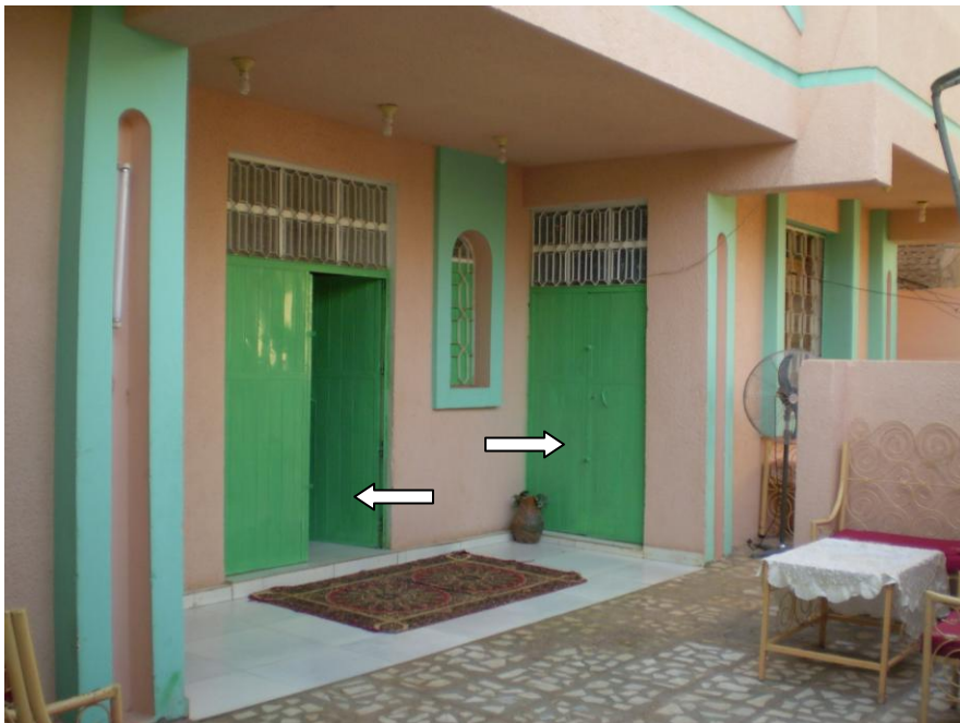
A double circulation leading from a courtyard into different sections of a house in Khartoum, Sudan
