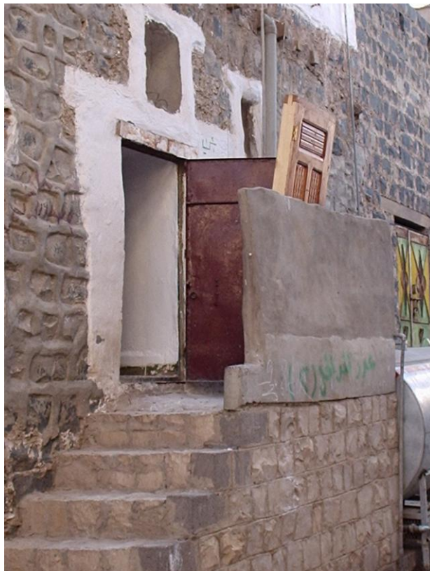
A wall placed just outside a front entrance for privacy protection in a house in San'a, Yemen.
