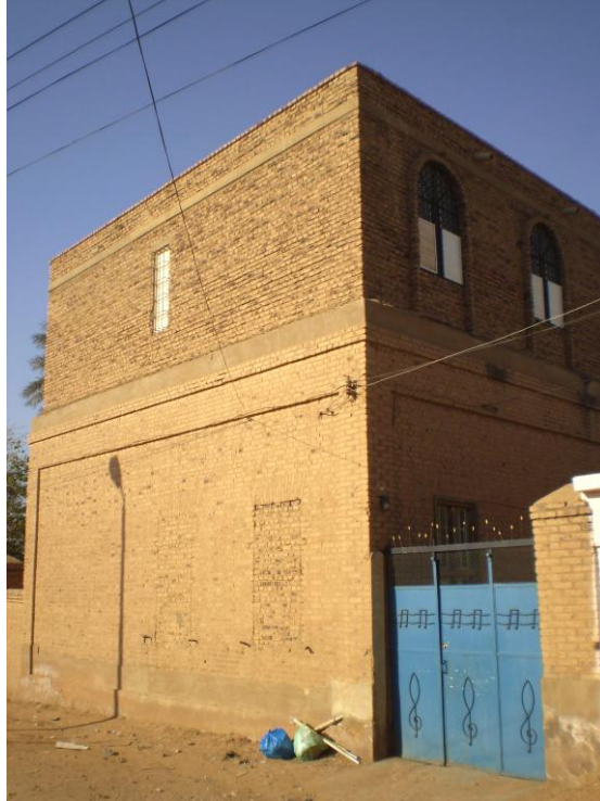
A house in Khartoum, Sudan. Windows are pierced in a façade which faces the house's courtyard, whereas the façade that faces a street and other houses across it, is virtually windowless.
