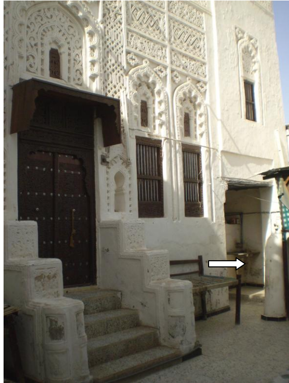
A separate entrance from a courtyard into a guest room, which adjoins a front door (pointed out), in a house in Zabid, Yemen.
