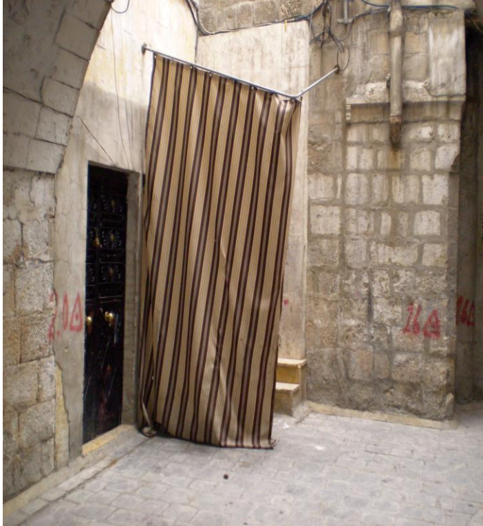
A crudely screened front entrance in a house in Aleppo, Syria.
